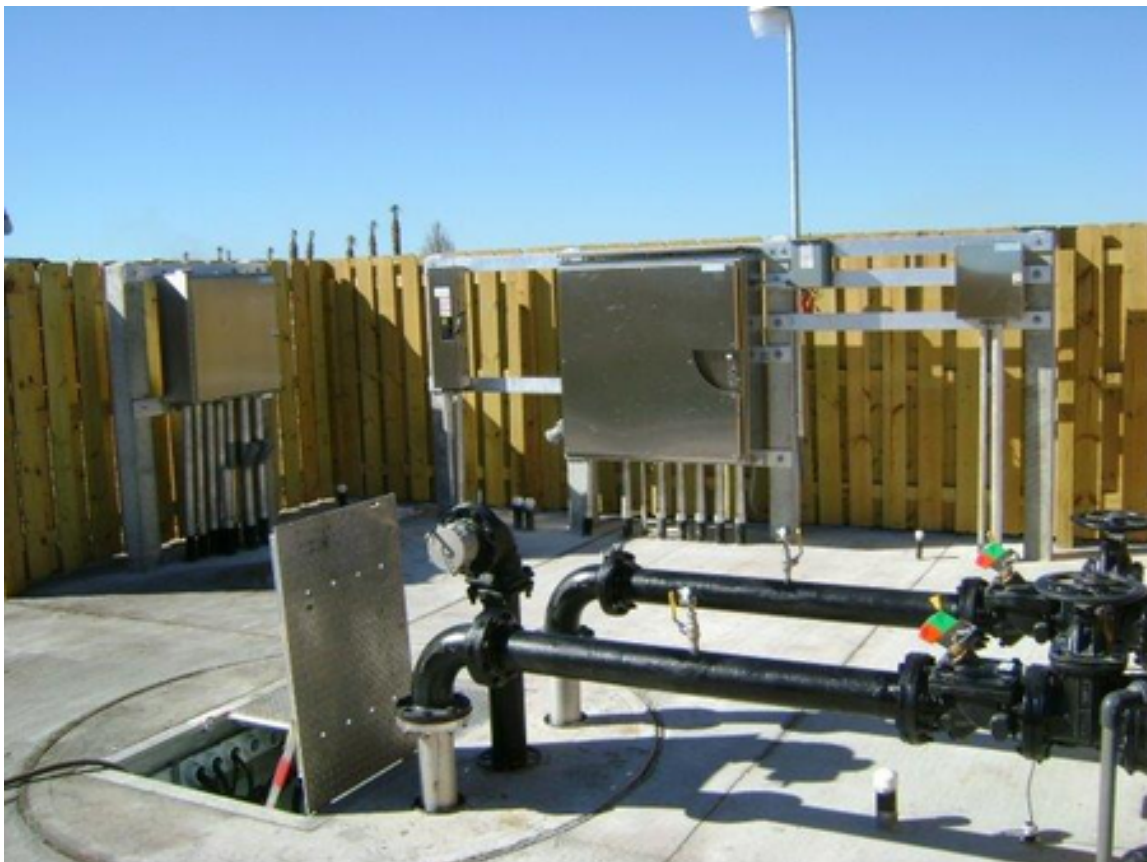
TOP EXTERIOR VIEW OF LIFT STATION
